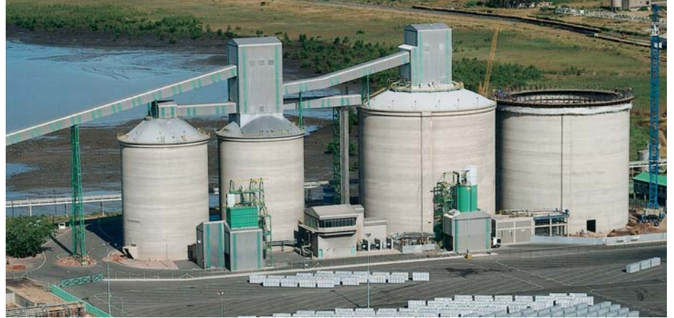
Mozal's raw material silos at the Matola Port
