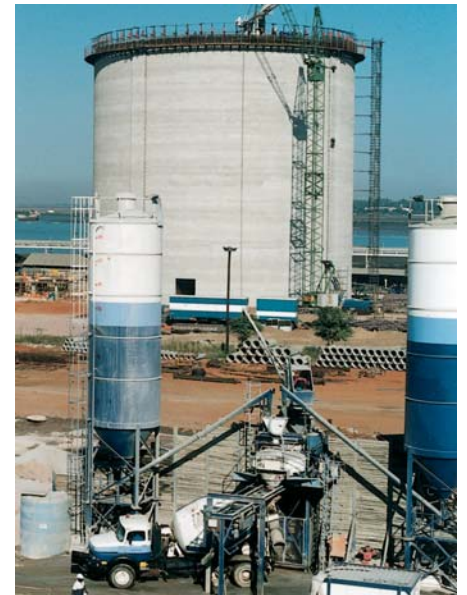
Below: On-site batch plant using OPC and Dura-Pozz®
