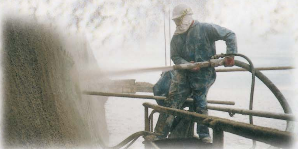
Wet sprayed concrete
